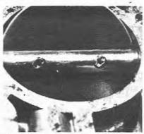
9.4a Main assembly: the butterfly screws have been bent over
